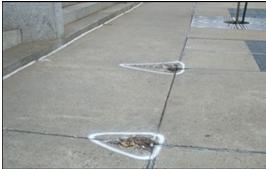
Areas of missing concrete have been identified for repair.
