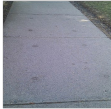
These panels were mud-jacked more than 20 years ago and are still in good condition
