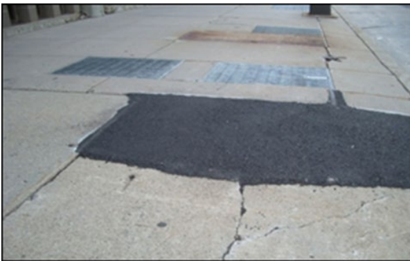
Wedge has been placed to mitigate the hazard caused by a raised sidewalk slab. Note the extensive and appropriate ramping of the wedge.
