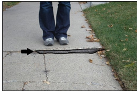
A small wedge may still create a hazard or be difficult to navigate in a wheelchair. This wedge had deteriorated over time.
