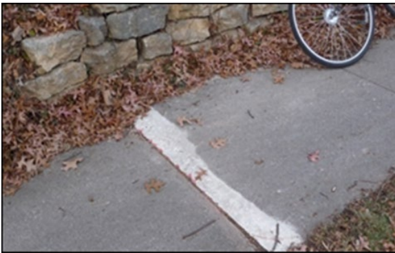
A raised sidewalk block has been ground down to provide a smoother transition.
