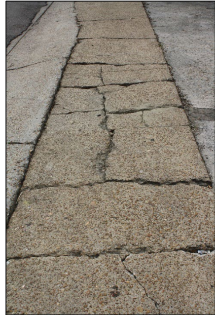
Cracking can cause trip hazards for pedestrians and wheelchair users.
