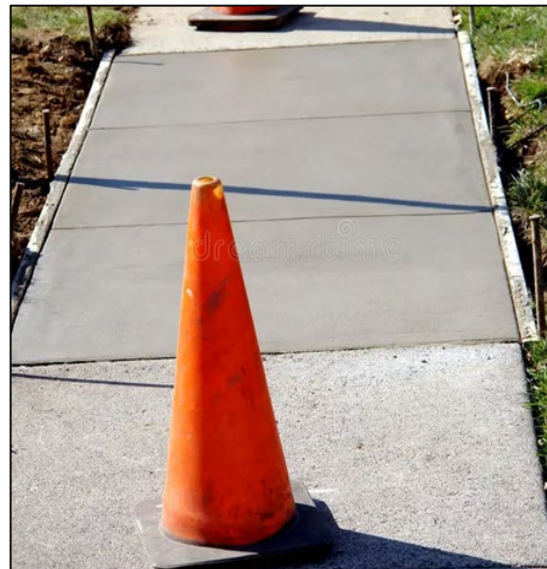
Sidewalk concrete panel replacement.
