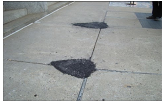
Affected areas have been temporarily fixed using asphalt patches. Note that the patching material covering the concrete extends beyond the perimeter of the hole.
