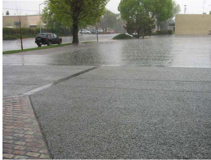
*Pervious Asphalt and Concrete Pavers*
